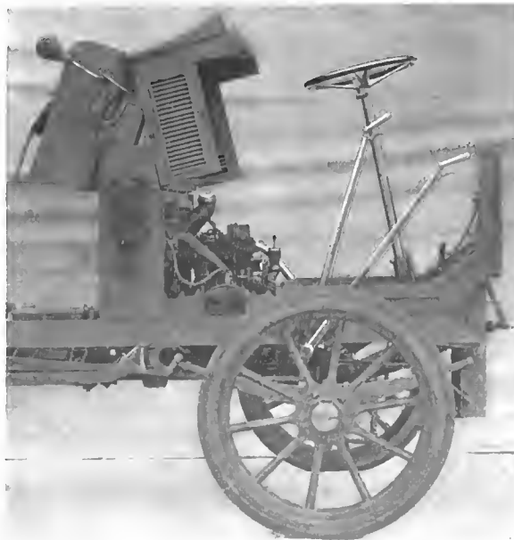
Showing the Accessibility of the Autocar Power Plant.
